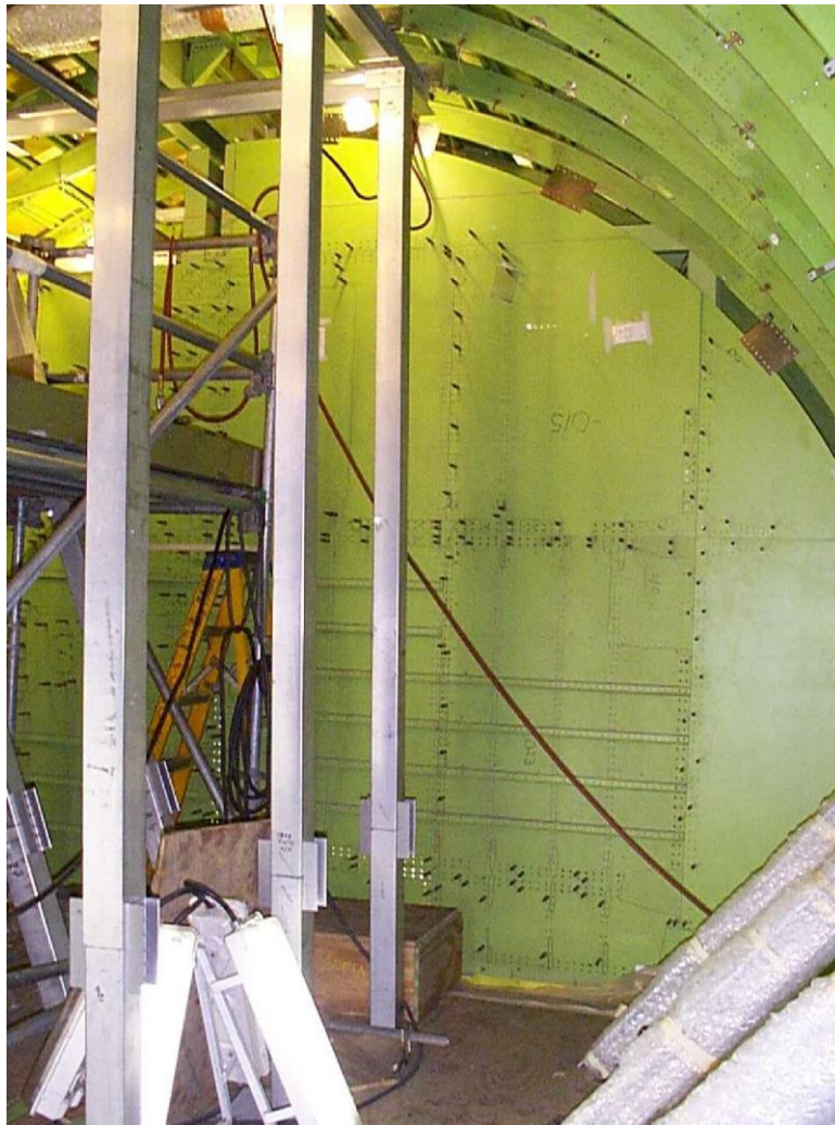
Figure 7.5-14. Aft bulkhead being installed into aircraft, Waco – October 2000.
