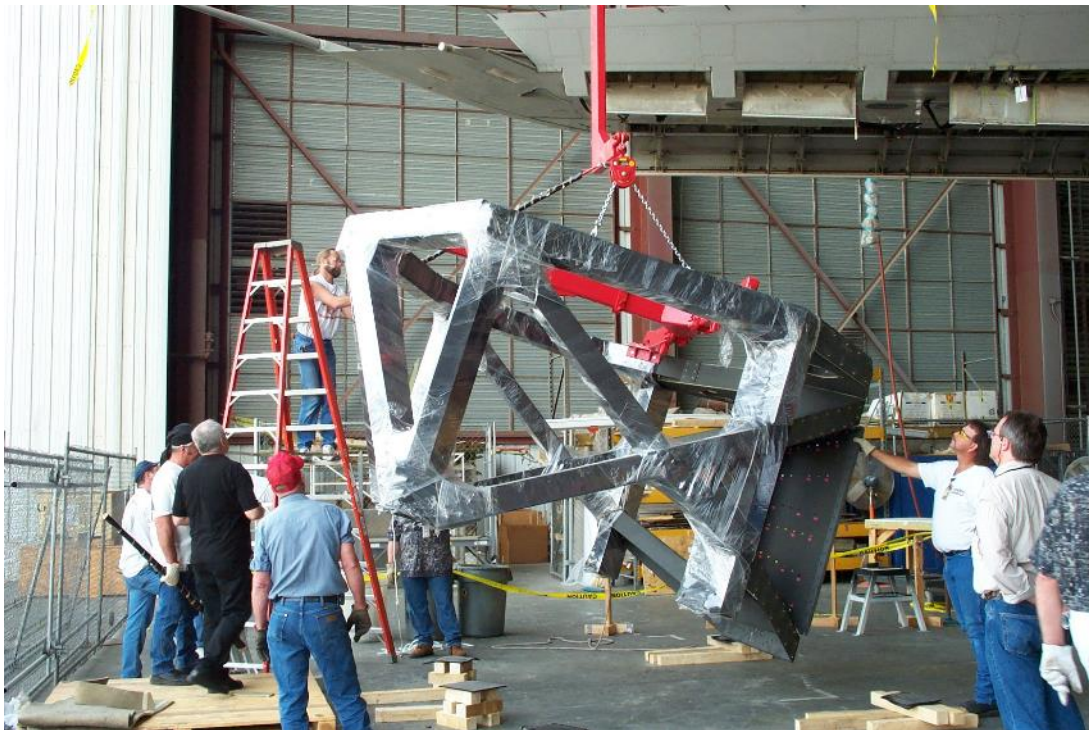
Figure 7.8-15. Lifting the telescope carbon fiber metering structure to install into the aircraft cavity onto the SUA – May 2, 2003.
