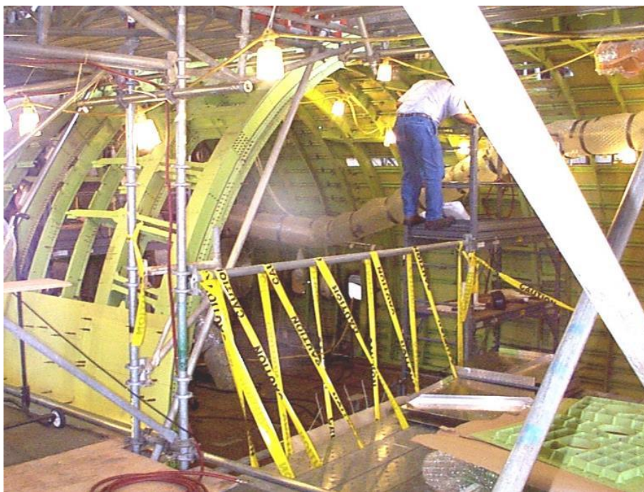
Figure 5.3-9. Looking into cavity opening from outside the aircraft.
