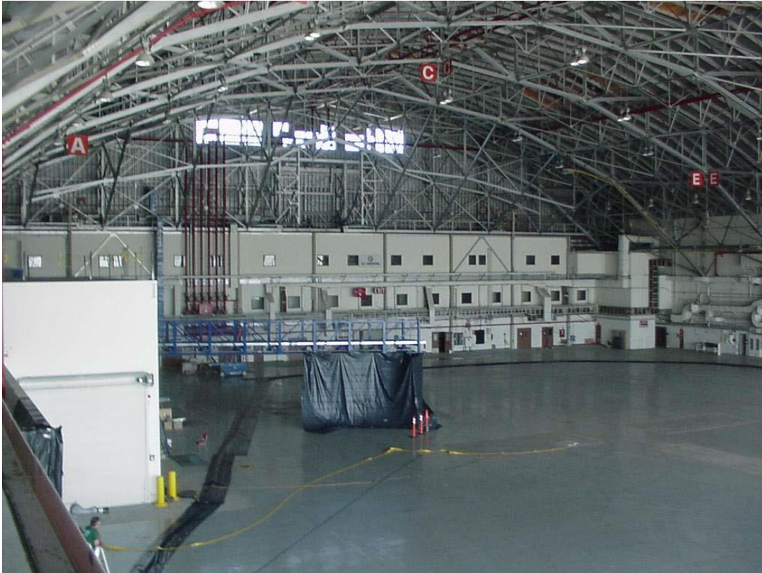
Figure 7.6-17. Inside of the N211 Hangar at Ames – June 2001.
