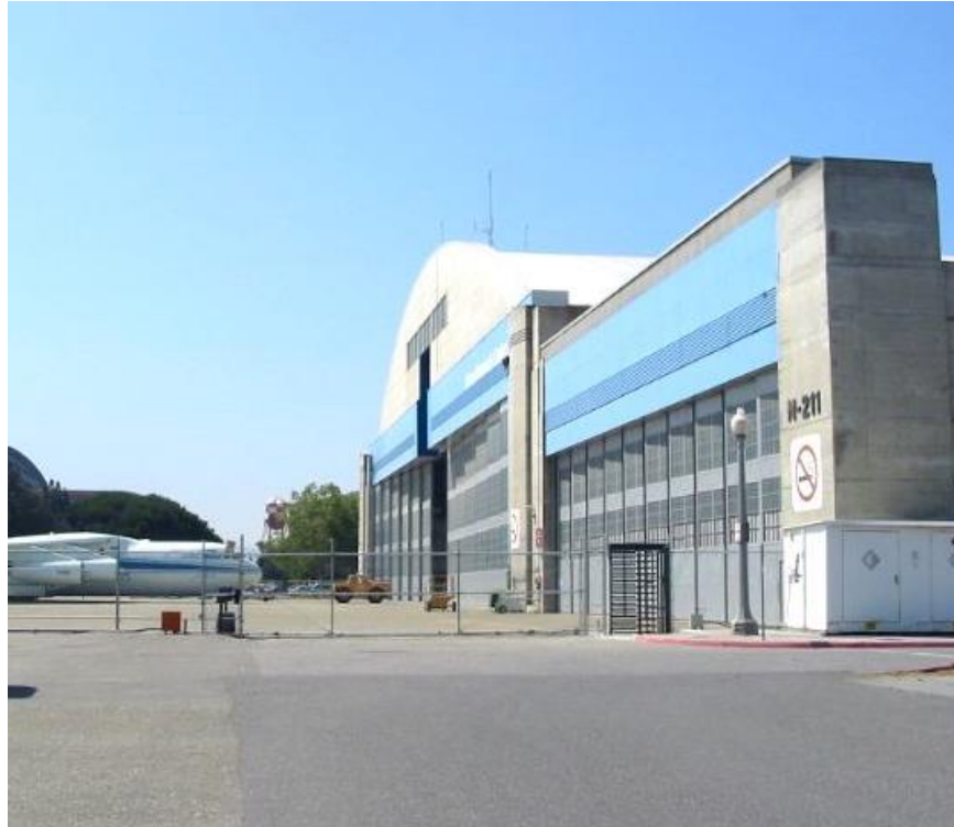
Figure 7.8-19. The outside of Hangar N211 at Ames showing the large notch modification installed above the door to accommodate the tall tail of the 747SP.
