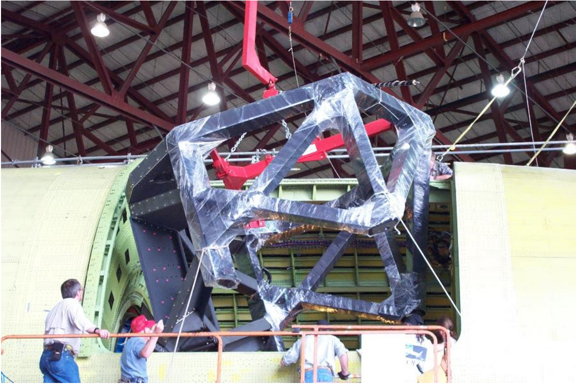
Figure 7.8-16. Lowering telescope metering structure into the cavity – May 2, 2003.
